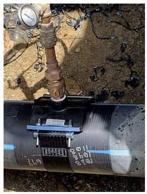
8" X 1" EF Saddle Pressure Tested Before Tapping
