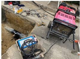
Typical Tooling Required For EF Saddle Installation
