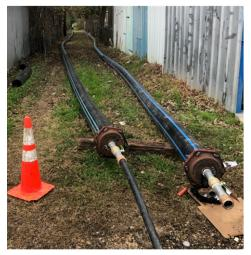
Hydro Static Pressure Test Prior to HDD/Bursting Installation
