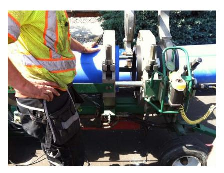
14" Butt Fusion/MJ Joint Adapter Fitting
